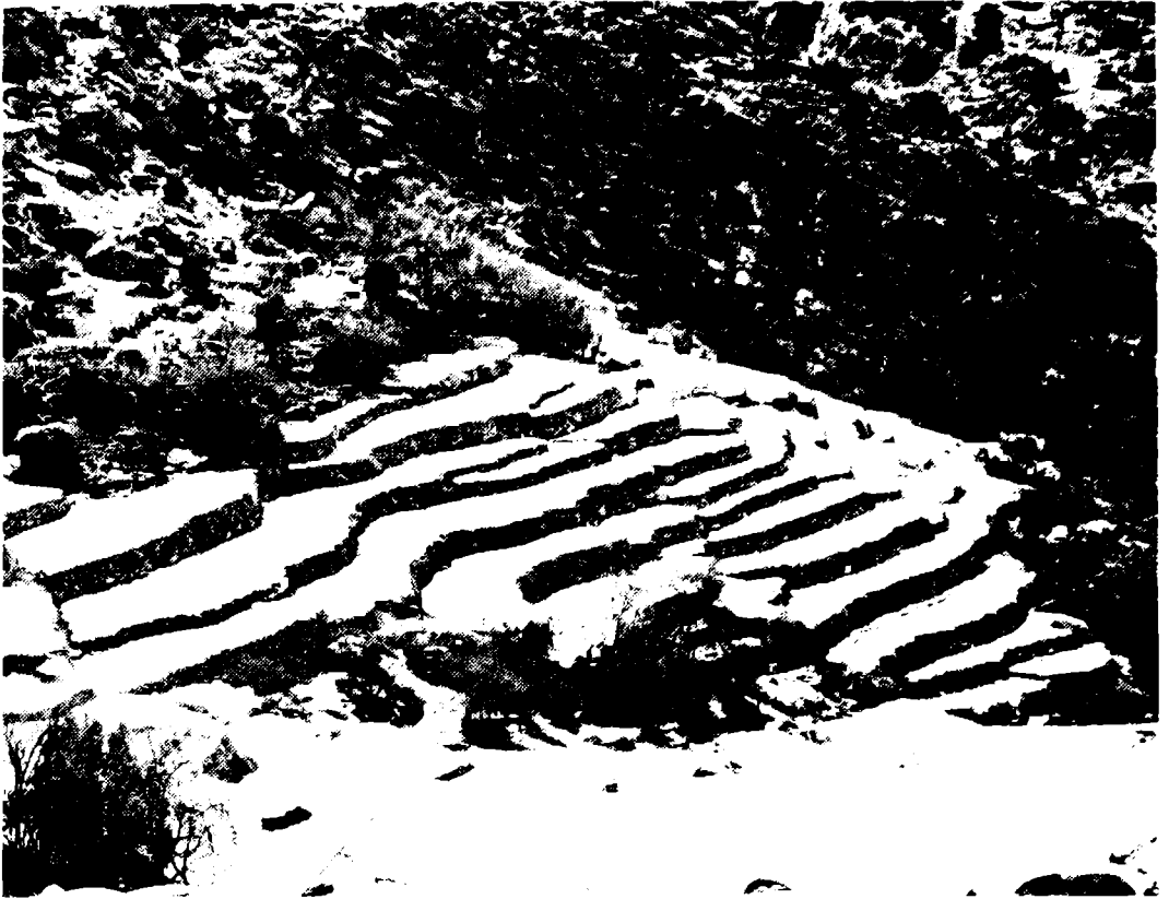
Terraced fields at Malil. Each terrace belongs to the man who constructs it, though in fact the job requires the work of several men, usually close agnates. The walls pictured here are 4-6 ft. high. The primary irrigation channel enters at the top where its course is marked by an uneven row of fruit trees. (Jan. 1961).
